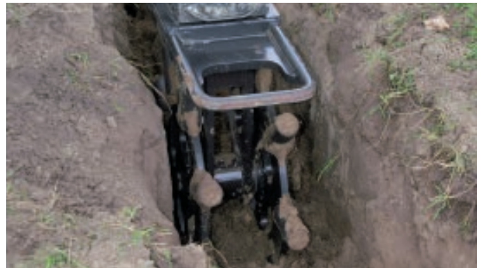
PACKER WHEEL – compact soil to spec after backfilling with this mechanical wheel
